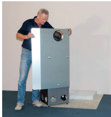
Fit the fire protection on the fireplace insert (special accessory). (2)
